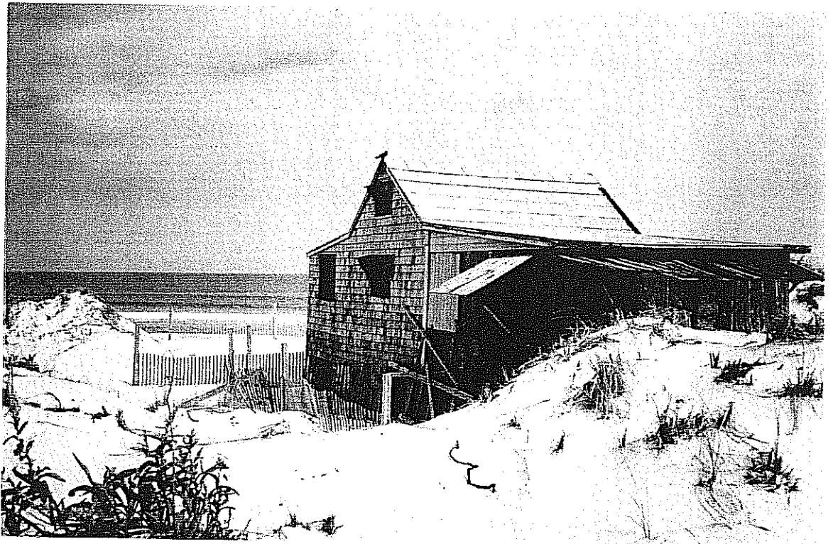
By the fall of 1997 the shack reshingling was complete, and the first of the porch repairs done. Note that the dunes facing the ocean had eroded over the last four years.
